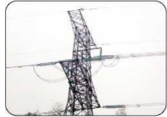
Electric power system
